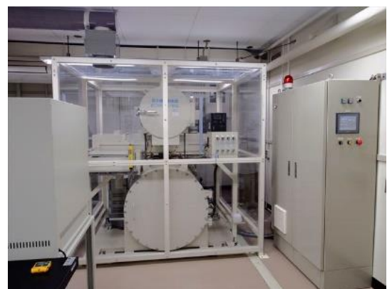
Fig.4 Exhaust booth around the electron beam accelerator for oxygen deficiency prevention
